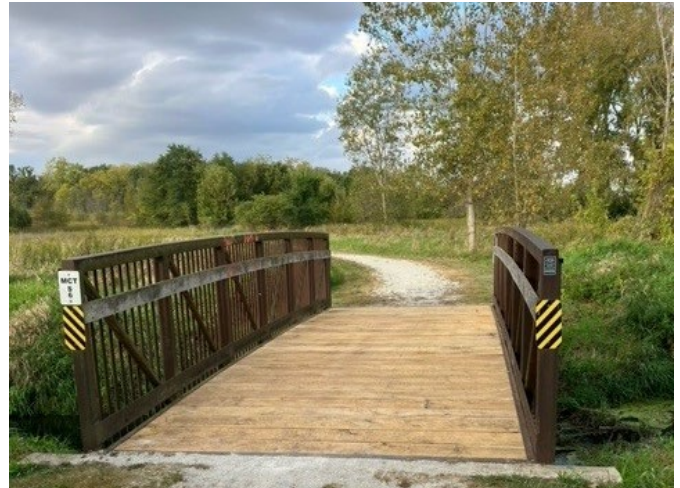
Operations staff completed a full replacement of the decking on the Virgil Gilman Trail bridge through Aurora West.
