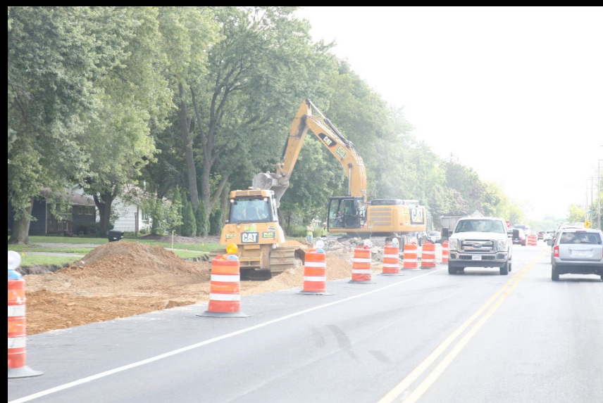
Crews break up and remove the old pavement on the Fabyan Parkway at Western Ave Intersection Improvement
