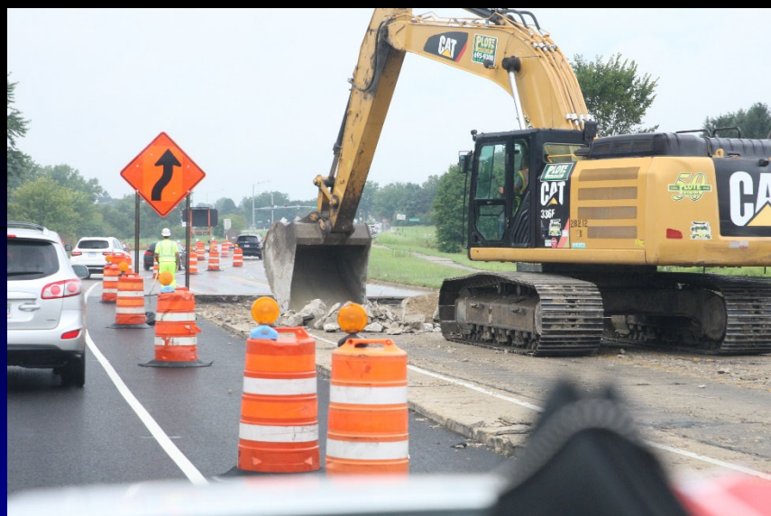
Crews break up and remove the old pavement on the Fabyan Parkway at Western Ave Intersection Improvement
