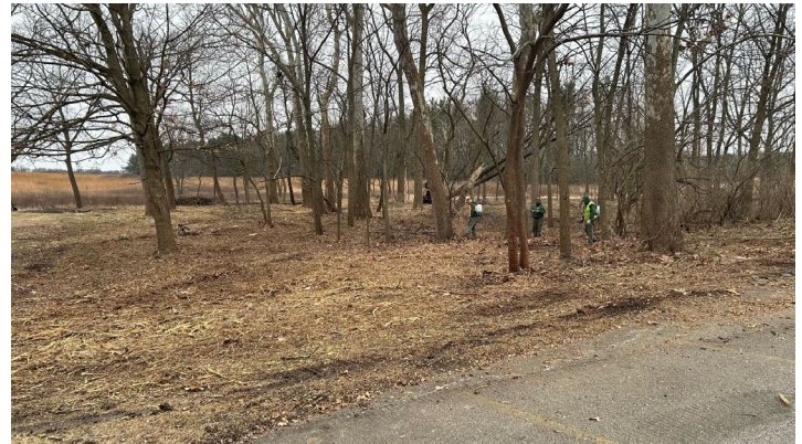
Tree clearing work done at LeRoy Oakes FP.
