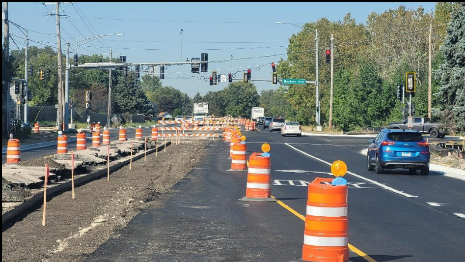
Crews work on base preparation, asphalt paving and new curb and gutter on the Fabyan Parkway at Western Ave Intersection Improvement
