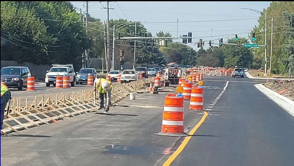
Crews work on base preparation, asphalt paving and new curb and gutter on the Fabyan Parkway at Western Ave Intersection Improvement
