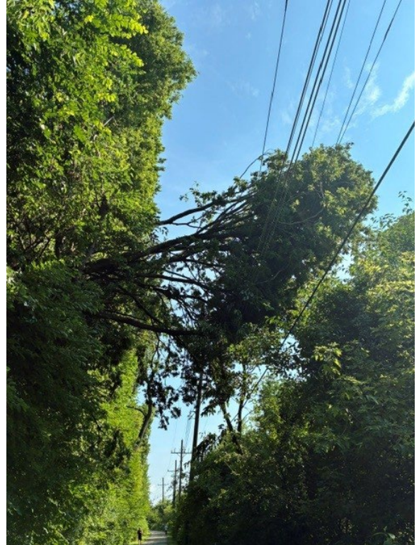
Trees downed during the storms fell onto utility lines along the Fox River Trail.
