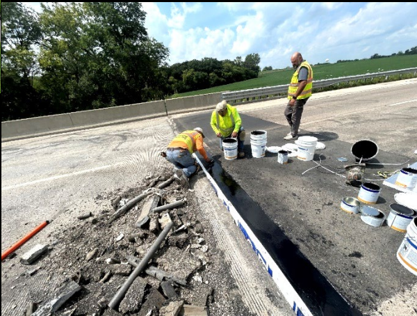
Crews complete removal and replacement of distressed pavement around expansion joints for the Claude Hansen bridge located on Randall Road over the UPRR in Elgin. The work will extend the life of the joints and provide a smoother ride for motorists. KDOT staff is working with the contractor on final quantities.
