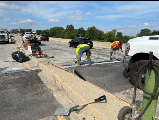
Crews complete removal and replacement of distressed pavement around expansion joints for the Claude Hansen bridge located on Randall Road over the UPRR in Elgin. The work will extend the life of the joints and provide a smoother ride for motorists. KDOT staff is working with the contractor on final quantities.
