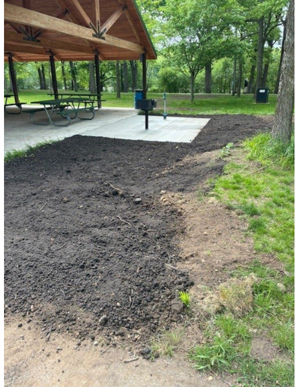
Concrete poured around both shelters at Jon Duerr FP.
