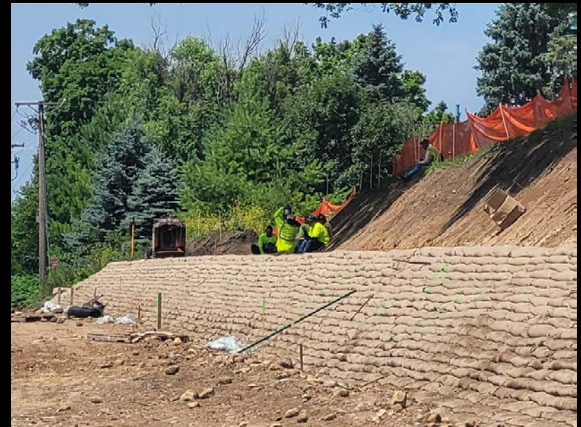
Crews continue work on roadway grading, storm sewer, curb and gutter and retaining wall installation for the new roadway alignment on the Bliss/Main/Fabyan Intersection Improvement project
