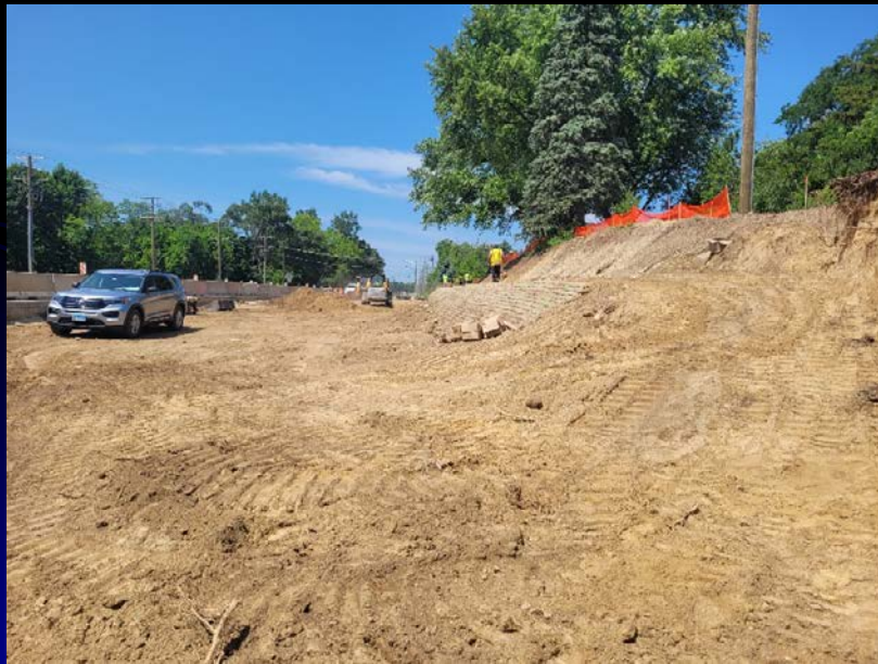
Crews continue work on roadway grading, storm sewer, curb and gutter and retaining wall installation for the new roadway alignment on the Bliss/Main/Fabyan Intersection Improvement project
