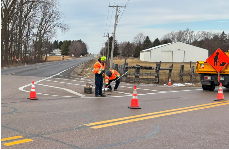
Stop bar on Burlington Road
