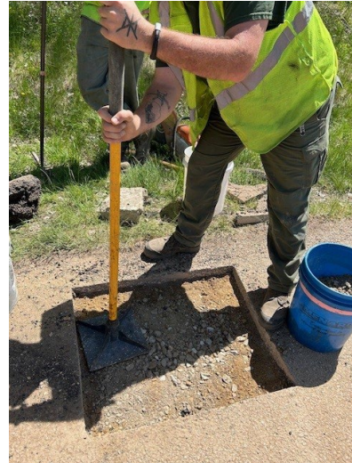
Pothole patching done along the Fox River Trail.
