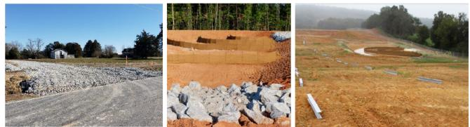
**Underground Work** (trenching for wires from PV combiner boxes to inverters, inverter pad installation, medium voltage cables to interconnection equipment)
