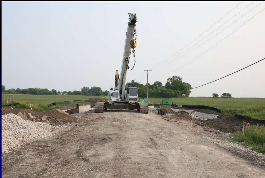
Crews work on grading and preparing road for new wearing surface as part of the culvert replacements for the Harmony Culvert Replacement project
