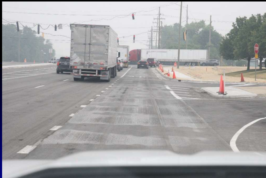
Diamond grinding crews work on eliminating bumps in the new pavement to improve the ride on the Orchard Road at US 30 Intersection Improvement project
