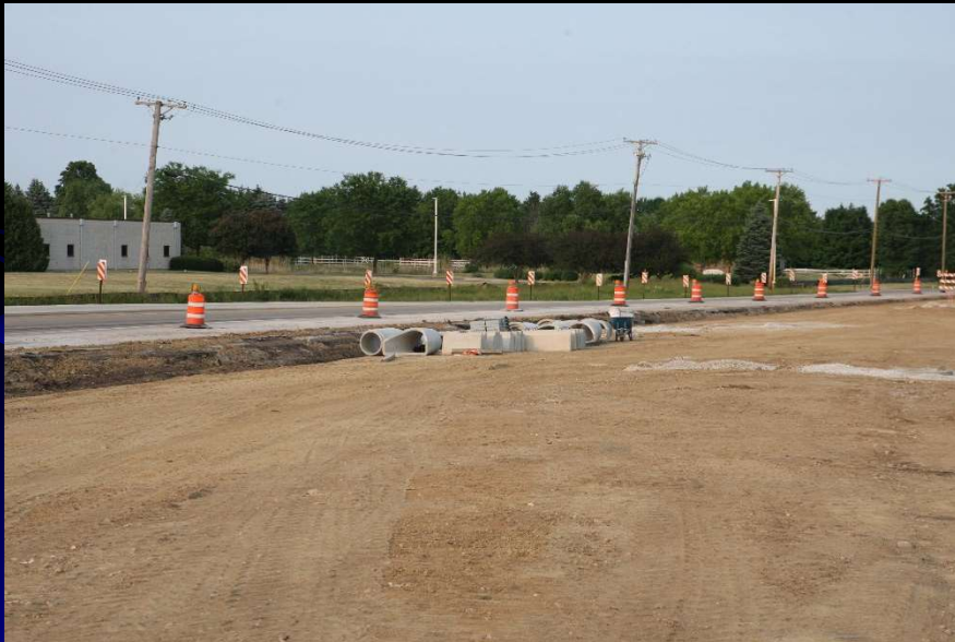
Crews work on excavation, storm sewer installation and grading for the new roadway alignment on the Bliss/Main/Fabyan Intersection Improvement project
