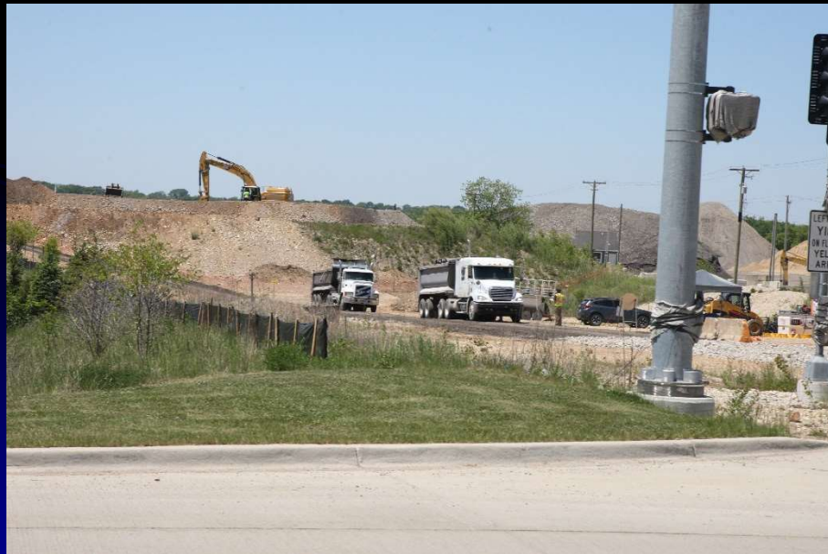
Treating, excavating, trucking, disposal and tracking of the contaminated soil keep crews at the LMP C-2A Soil Disposal project busy
