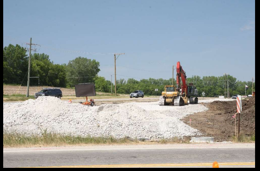
Crews work on excavation, storm sewer installation and grading for the new roadway alignment on the Bliss/Main/Fabyan Intersection Improvement project
