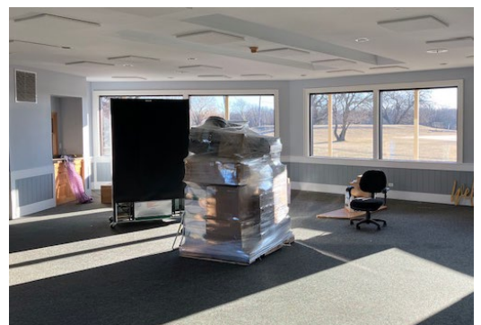
Working on repairs and maintenance at Hughes Creek Golf Course clubhouse.
