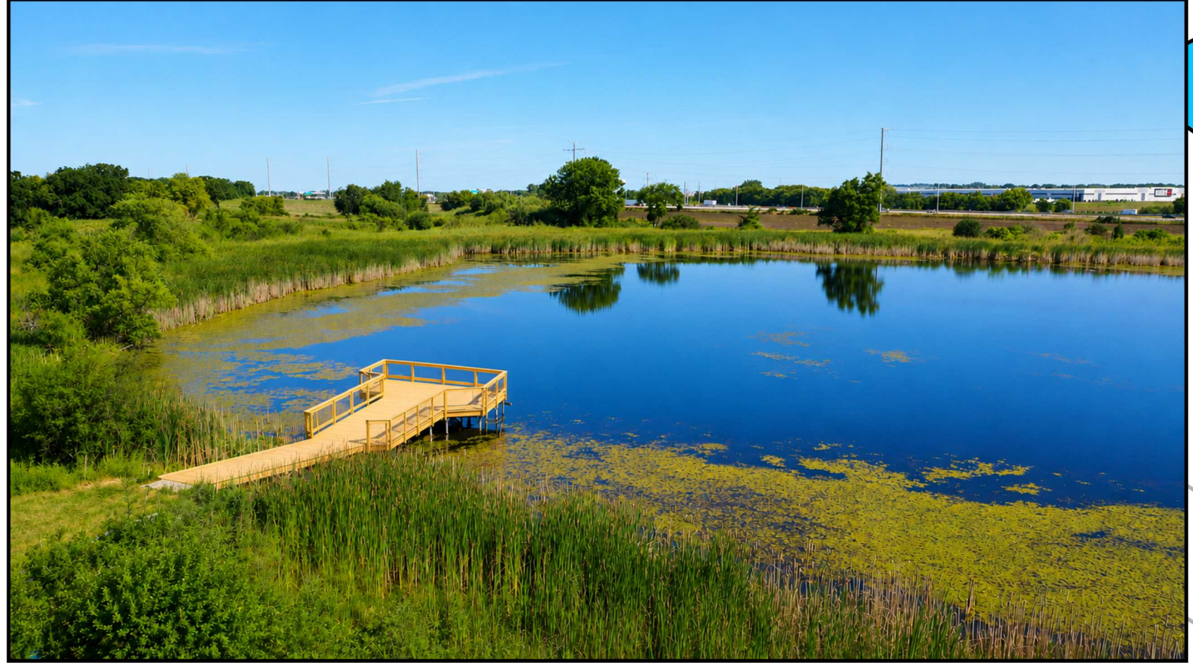
New Fishing Pier and Stone Outcropping Areas
