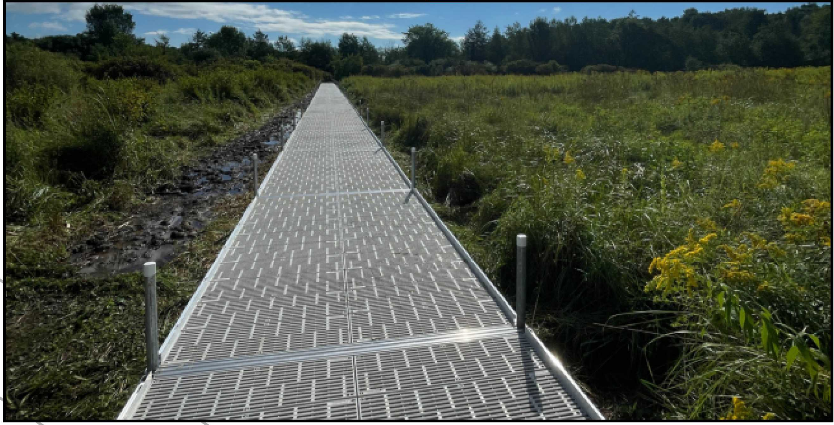
New Low-Profile Metal Grate Boardwalk on Steel Pilings
