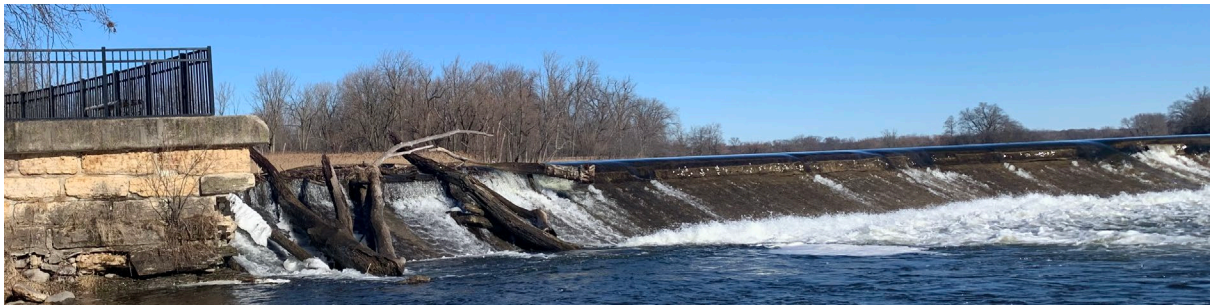
Carpentersville Dam, February 2023
