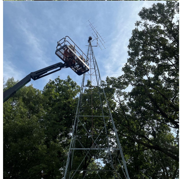
Photos of the MOTUS tower being installed at Needham Woods.
