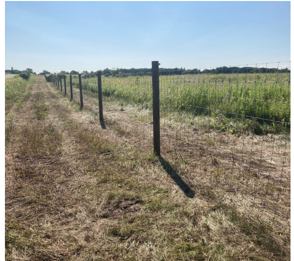
First phase of bison fencing construction completed at Burlington Prairie FP.
