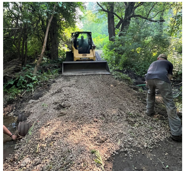
Staff laying down crushed limestone for trail repairs.
