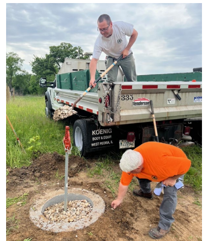
Crew Leader Smith and Ranger Technician Stoecklein putting finishing touches on a new water hydrant at Burlington FP.
