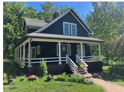
Photos of the new siding installed on the Fabyan FP staff residence.
