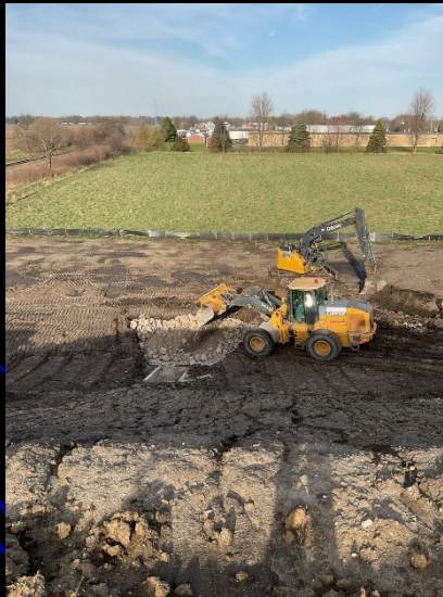
Crews work on bridge deck construction as well as drainage and site work on the Dauberman Road Extension project
