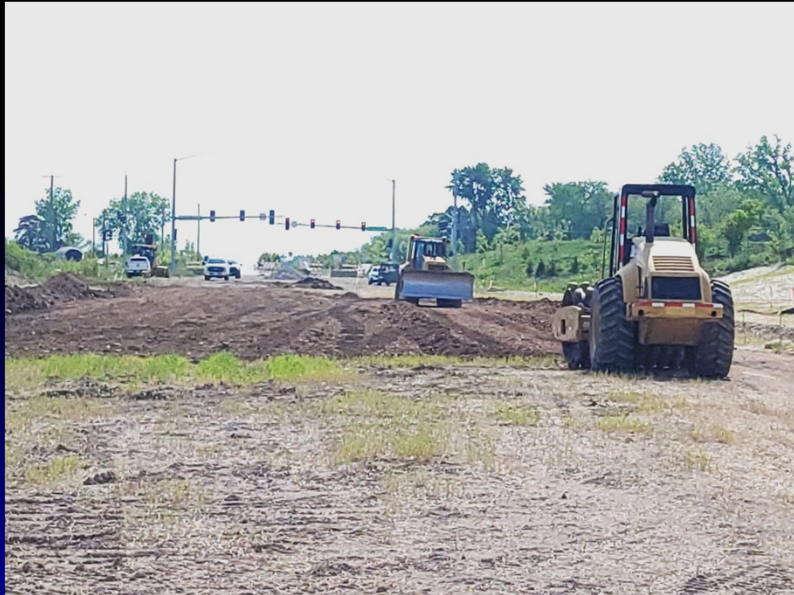
Crews work on erosion control, storm sewer installation and site grading on the LMP C-2B contract
