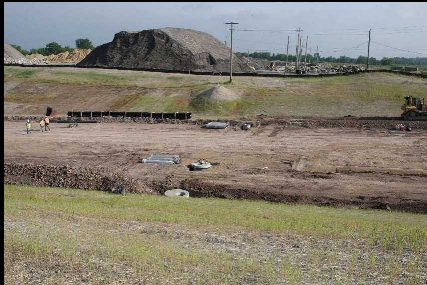
Crews work on erosion control, storm sewer installation and site grading on the LMP C-2B contract
