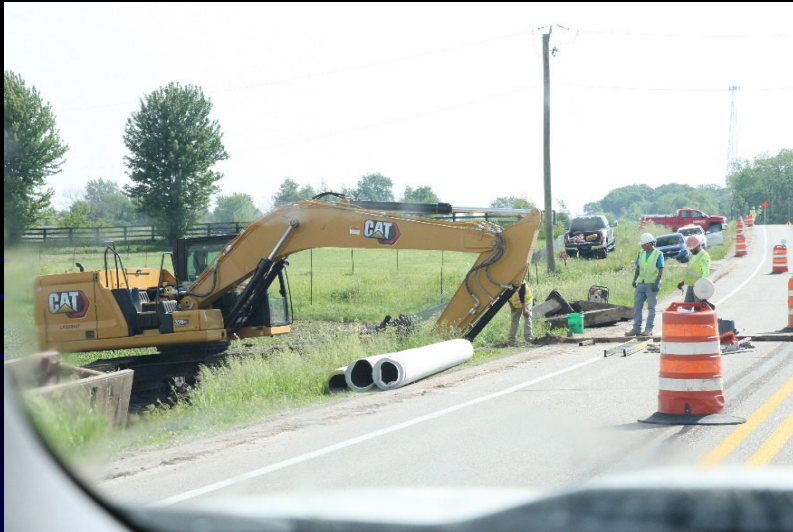
Crews work on installing storm sewer laterals on the Plank Road - Engel to Waughon HSIP project
